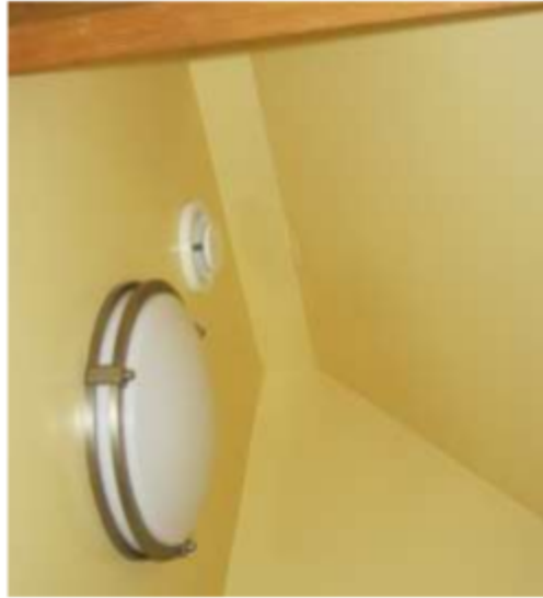
Figure 12: None of the flow hoods would fit into the space adjacent to this bathroom ERV inlet; it went unmeasured
