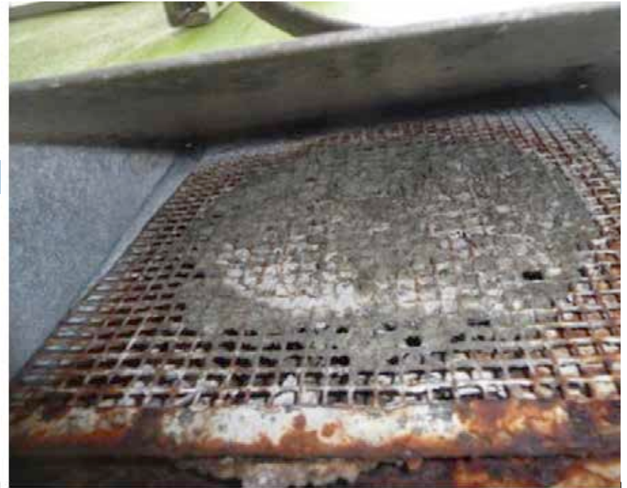
Dirty outdoor air intake.
