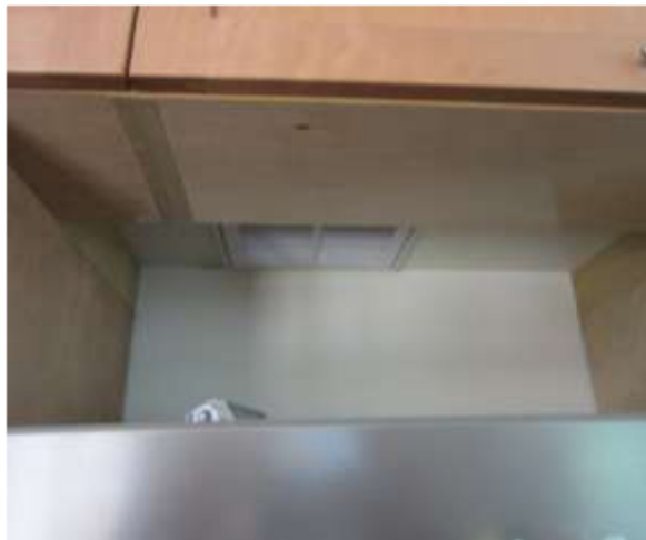
Figure 14: The refrigerator has to be pulled out to measure this kitchen ERV inlet, and even then, the uneven surface prevented measurement with most of the flow hoods
