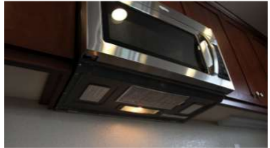
Figure 17: The dimensions and irregular surface of this typical microwave-integrated range hood in FH2 make inlet flow measurements difficult
