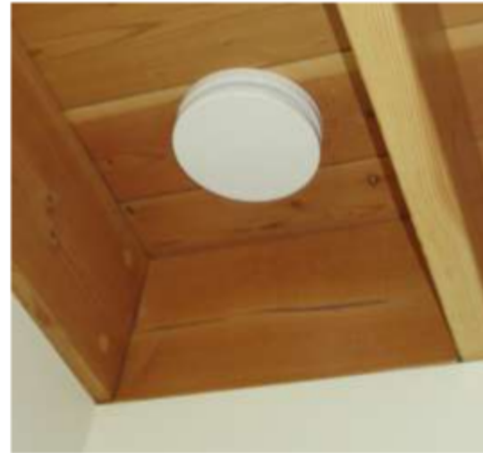
Figure 13: Only the smallest flow hoods could measure this ERV outlet set between floor joists
